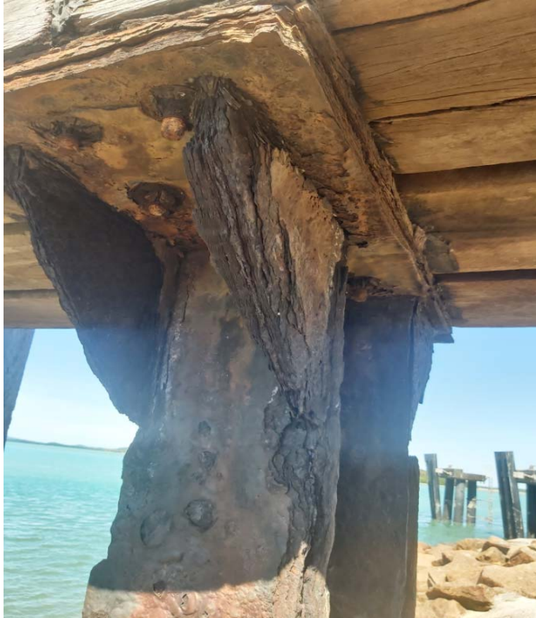
Photo 1 - Pile 'headstock' on Badu finger jetty - significant corrosion and delamination evident.
