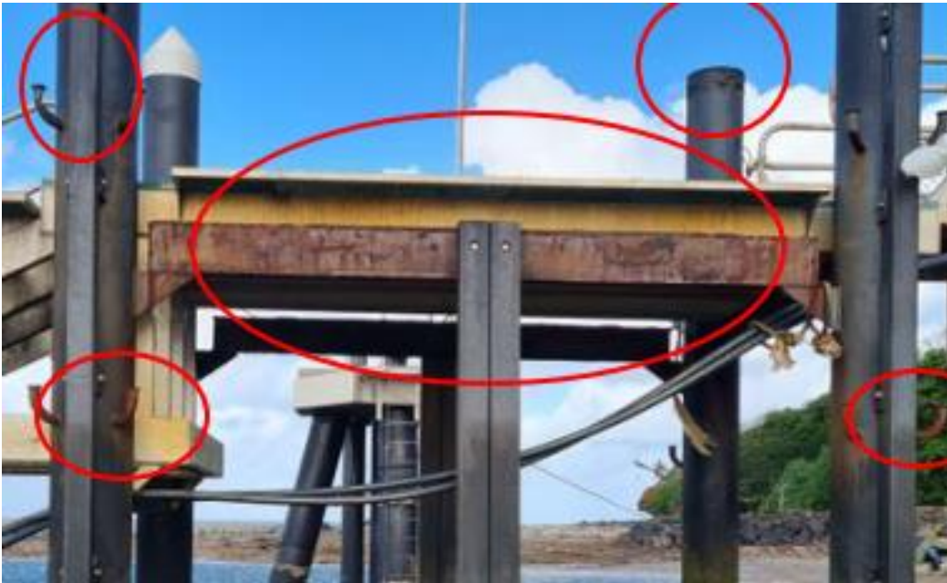
Figure 4: Longitudinal Beam requiring replacement
