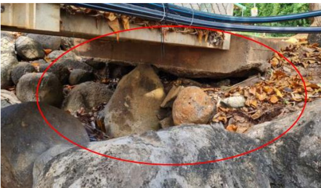
Figure 3: Undermined jetty access slab
