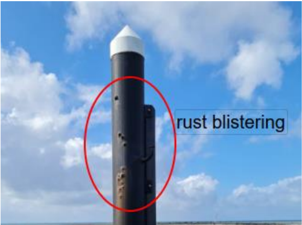
Figure 5: Rust blistering on marine pile
