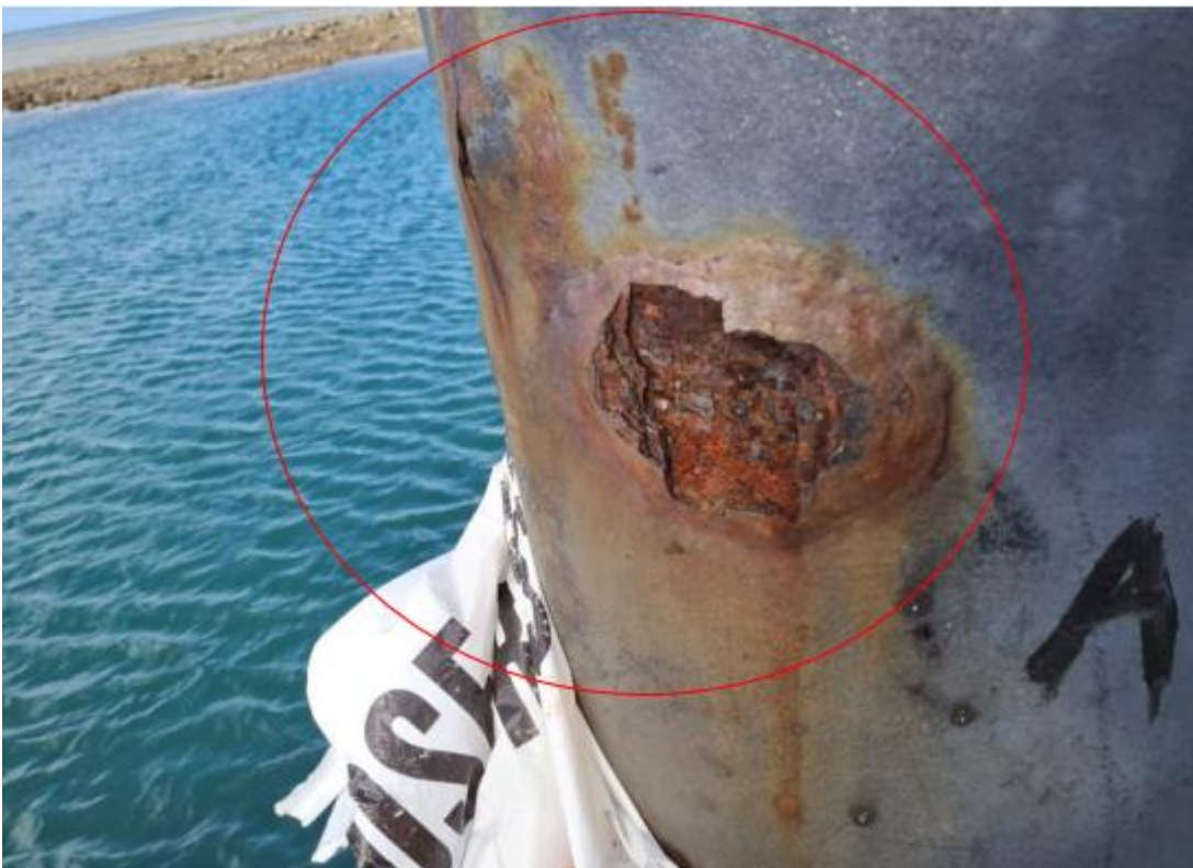
Figure 1: Mooring Hook completely rusted off
